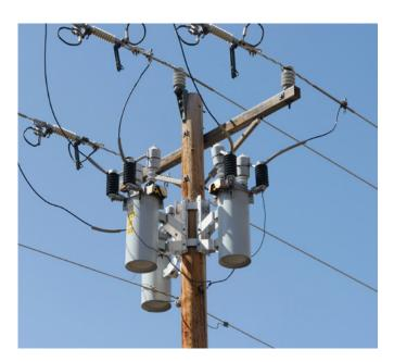
There are also recloser systems with inbuilt RTU modules which allow a high level of measurement capability as well as some control capability. There could be data logging and remote control functionality, full directional protection for overcurrent, earth fault and sensitive earth fault, over and under voltage, over and under frequency and auto reclosing functionality.
