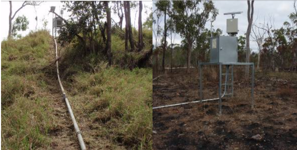
Figure 6 Pipe installation at Keelbottom Creek (left) and Scrubby Creek (right) both located on the Department of Defence Townsville Field Training Area. The pipe is attached to piers located on the downstream side and offers good protection against fire.
